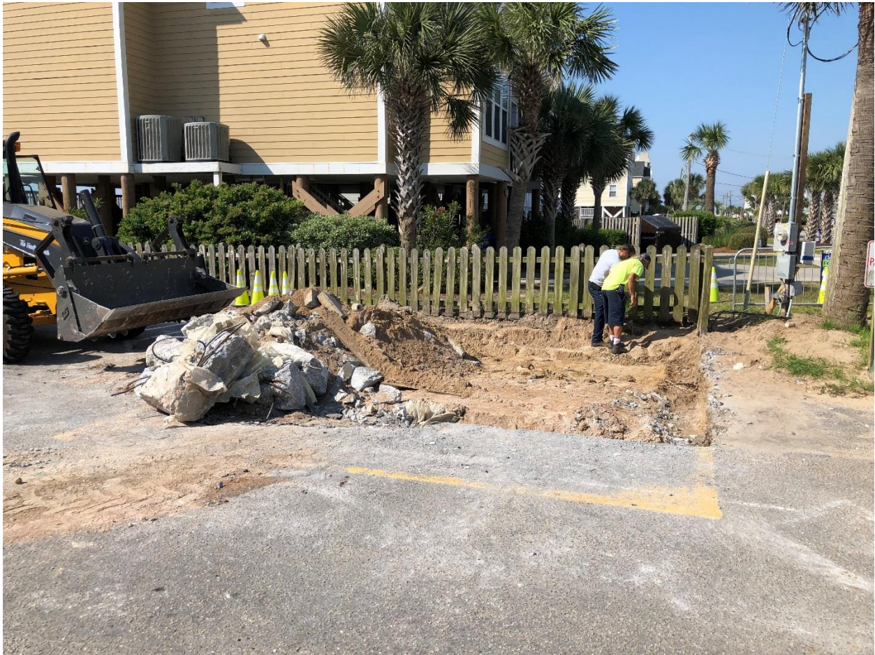
Site prep work for the new 13 th South Restroom
