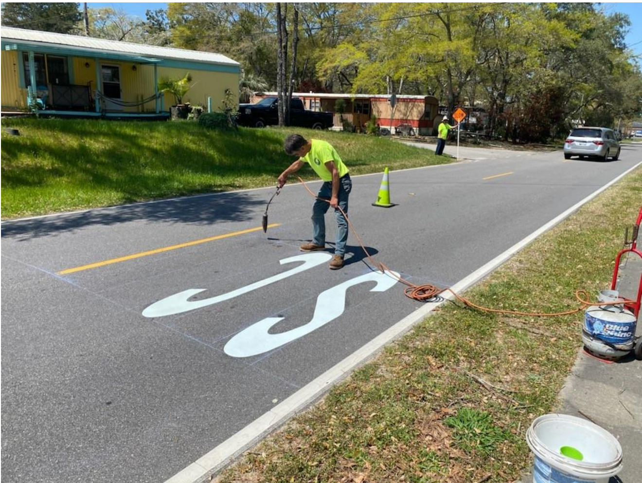
Crews install thermoplastic traffic warnings on 16 th Ave N.
