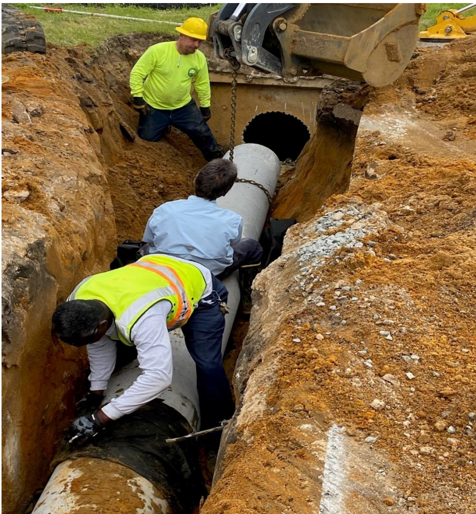
Poplar South Drainage Relief Line installation.
