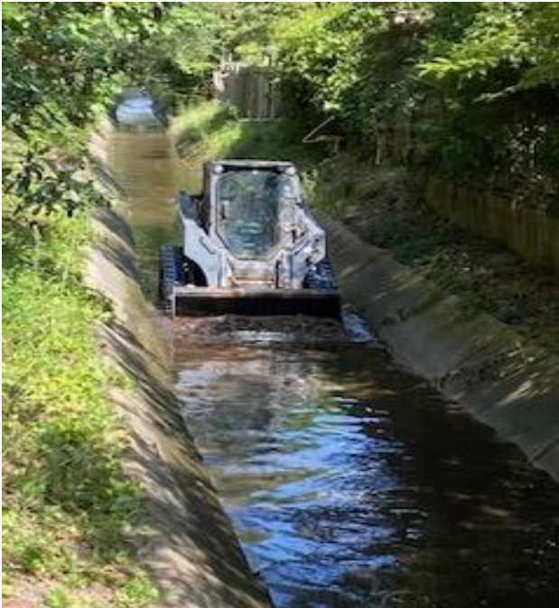
Canal cleaning off Lakeside Drive
