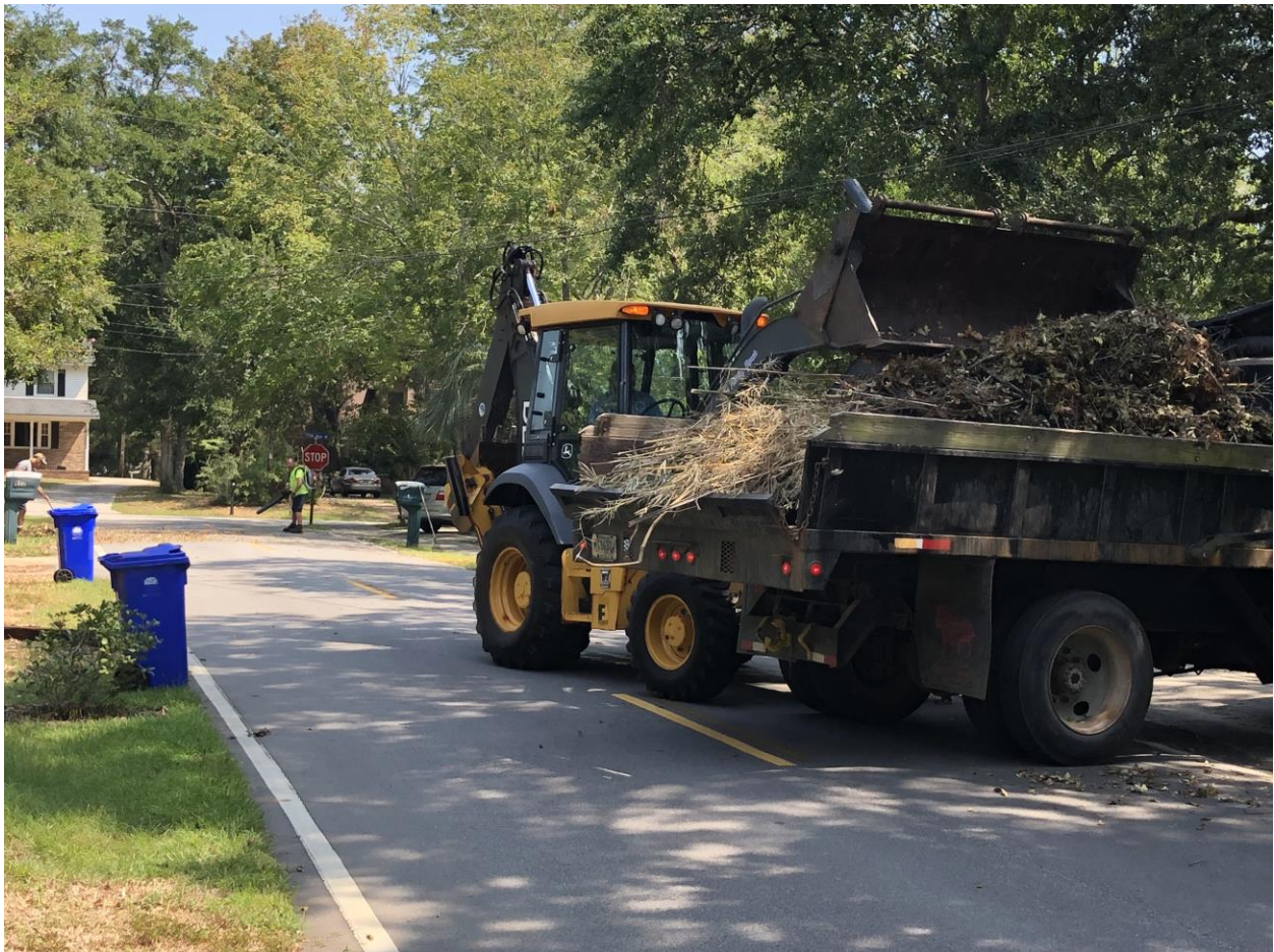
Crews remove vegetative debris generated by Hurricane Dorian
