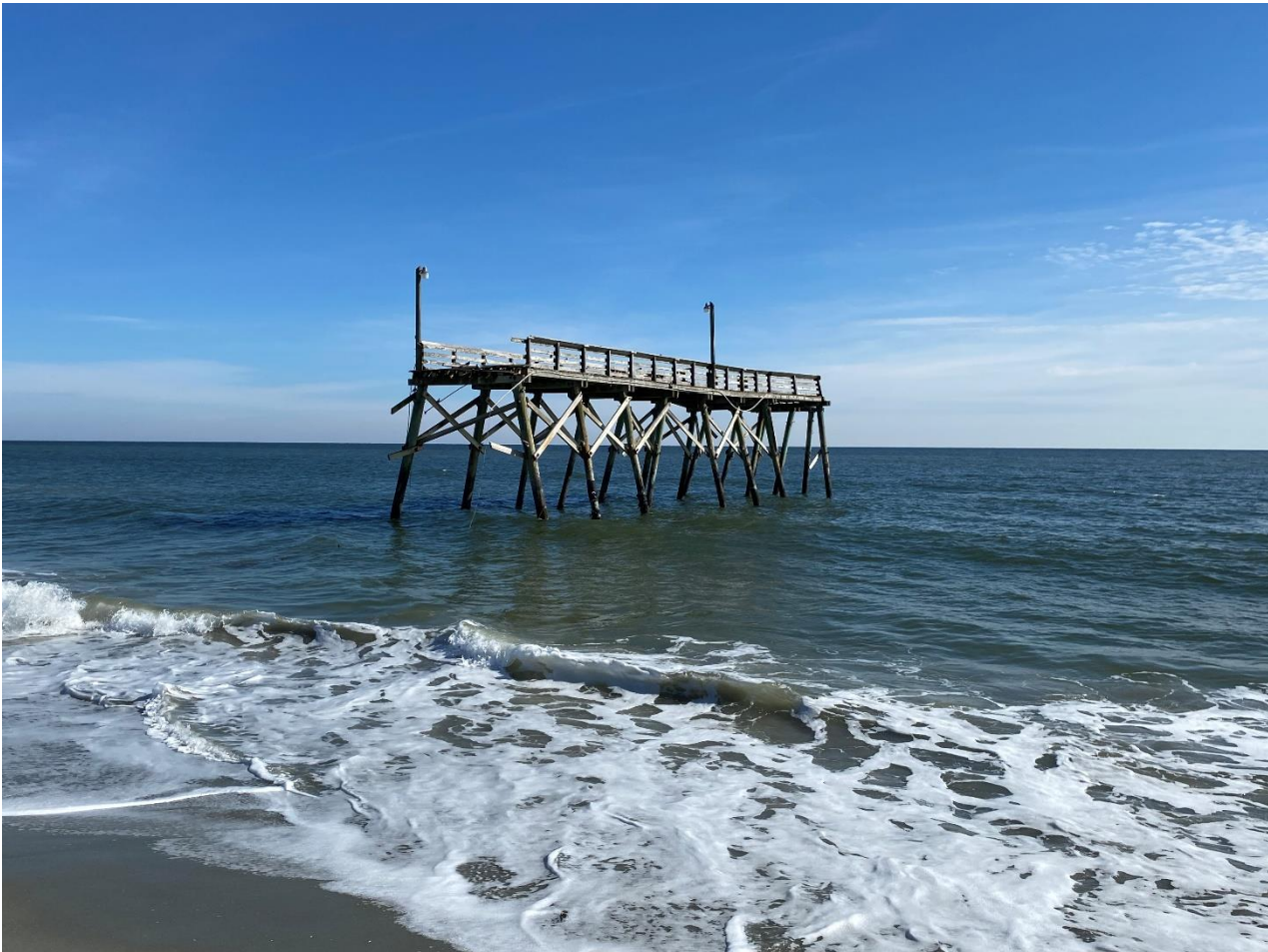
The end of an era! The final segment of the wooden Surfside Beach Pier stands defiantly, prior to final demolition on 12/10/2020.
