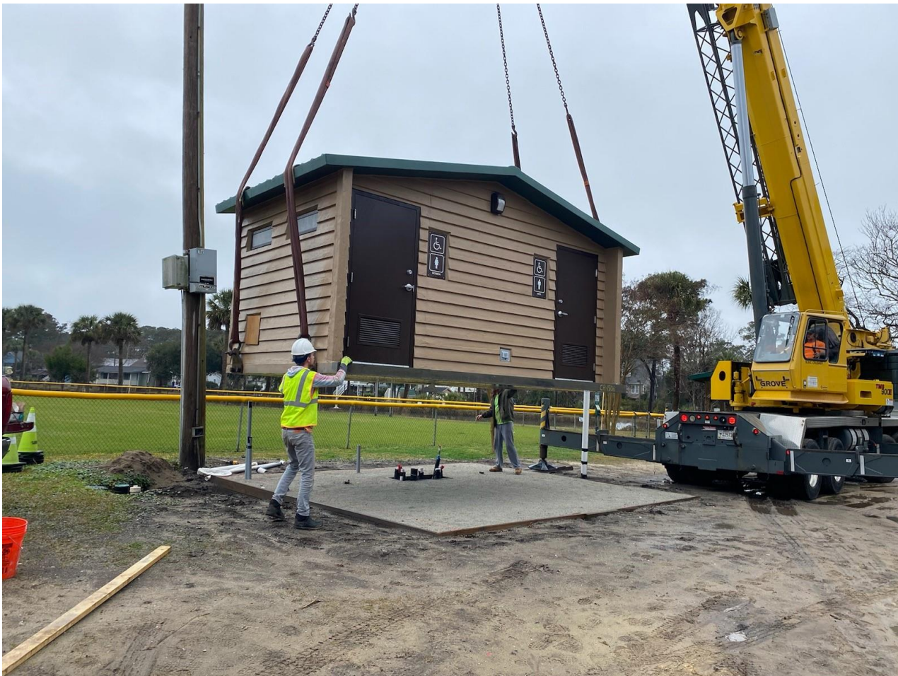
New, ADA-compliant public restroom delivery to Martin Field 1/27/21.
