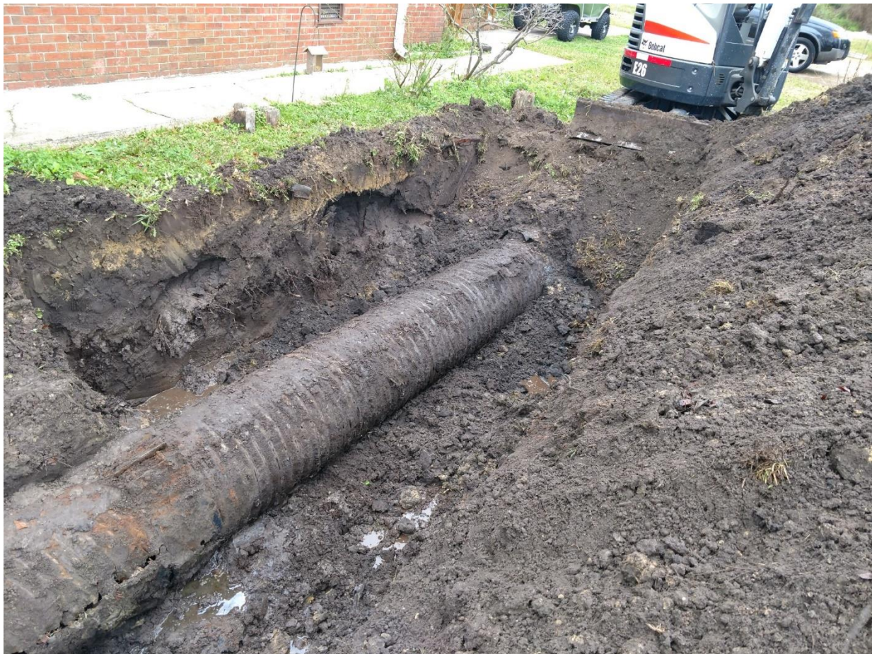
Drainage line replacement on Poplar Drive South – January 2020.
