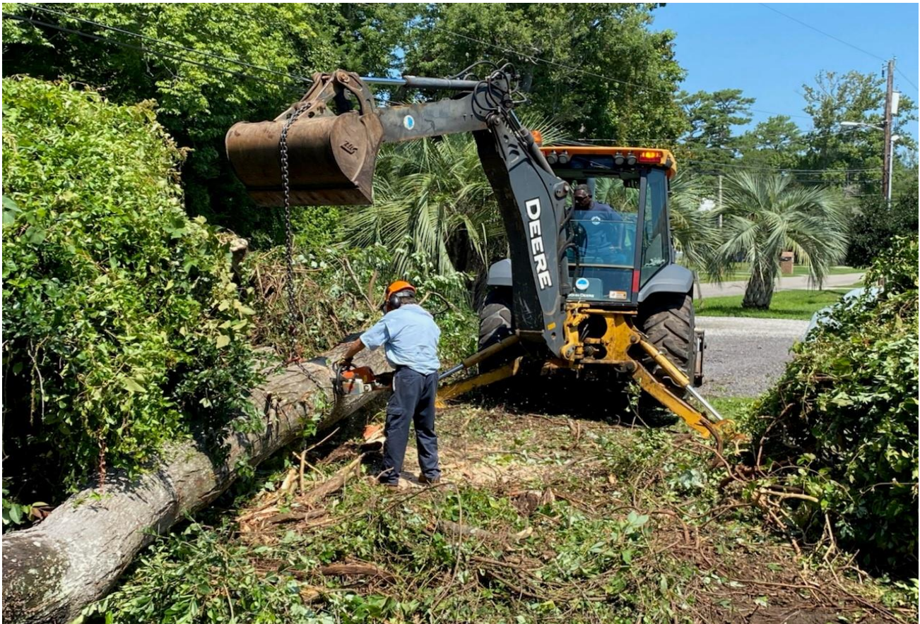
Crews remove downed tree from stormwater canal – 7/2020
