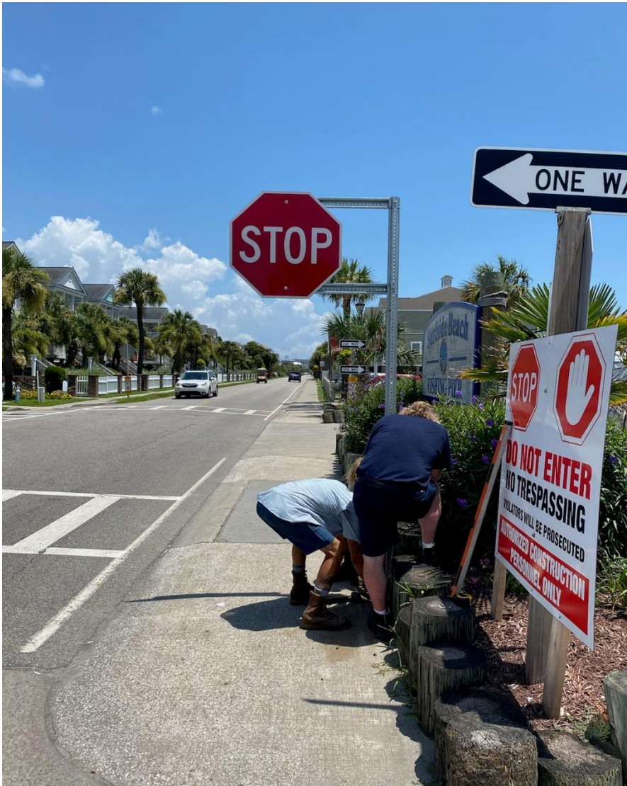
Crews install 3-way stop at Surfside Drive And Ocean Blvd. 7/16/21.
