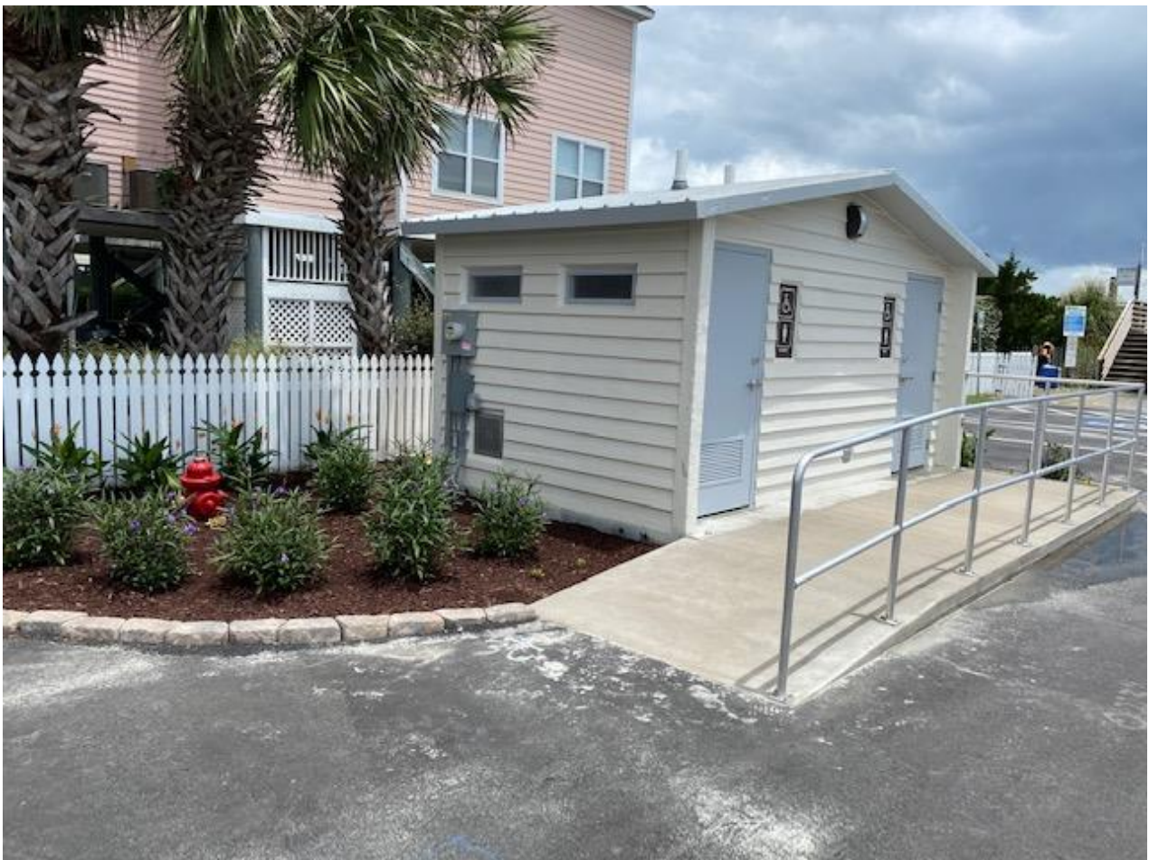
New Beach Restroom at 3 rd Avenue North Lot.
