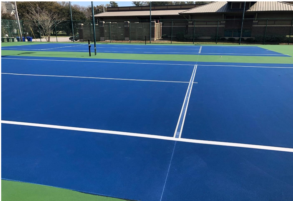
March 2020 Tennis Court resurfacing
