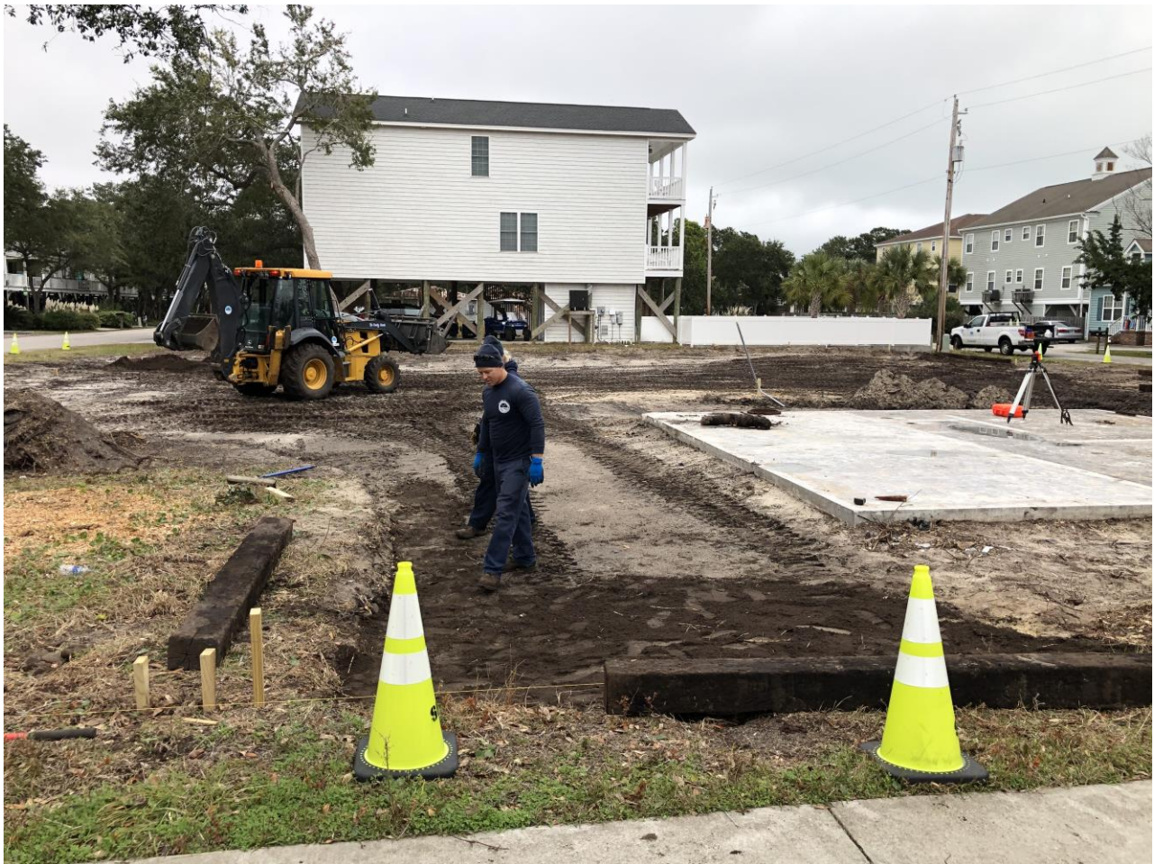
Crews preparing new parking lot for use.
