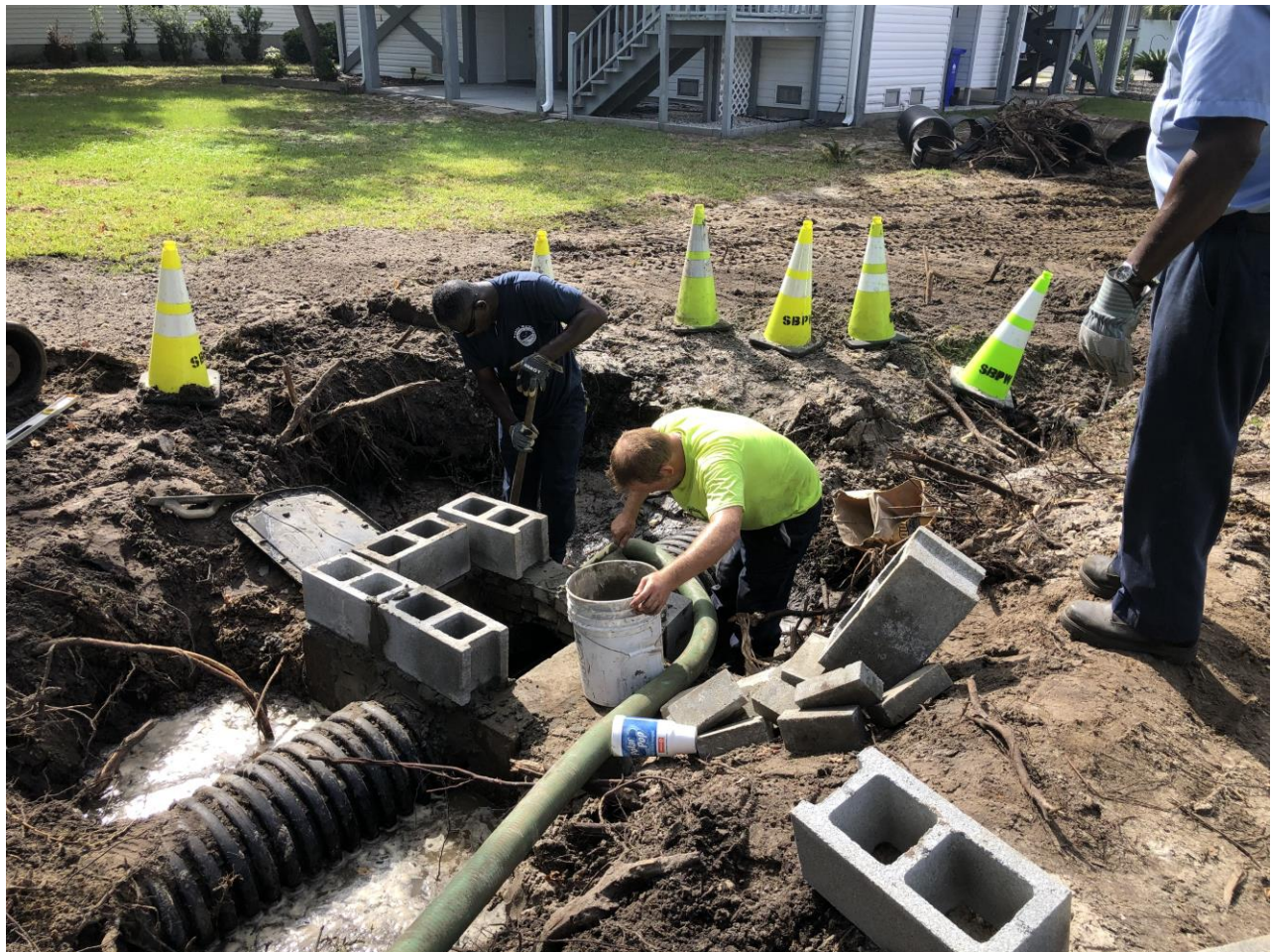
Crews perform drainage easement repair on 16 th Avenue North.
