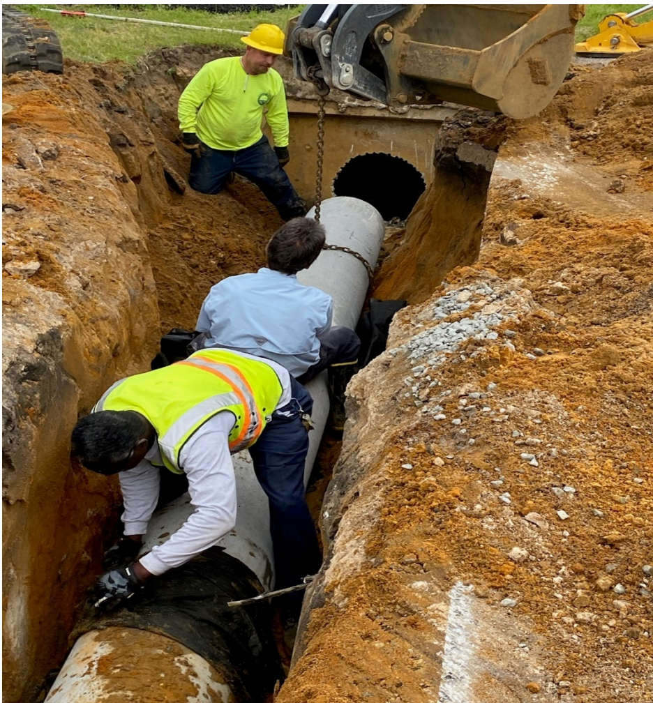
Poplar South Drainage Relief Line installation.
